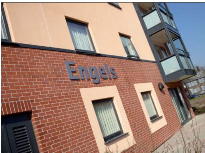
Fastbrick on ground floor with Silicone render detailing around windows
